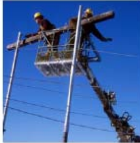
Contractors Constructing the Mayo-Dawson Transmission Line ( www.archbould.com )
