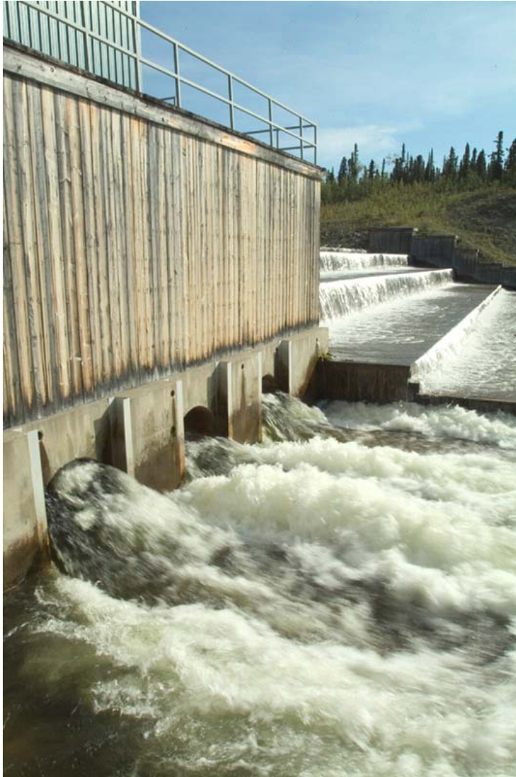
Mayo Lake Control Structure ( www.archbould.com )
