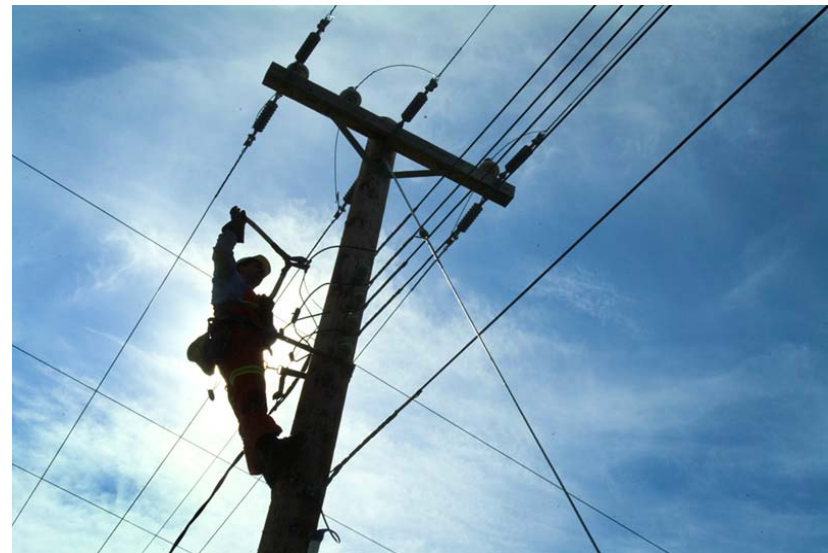
Line Maintenance ( www.archbould.com )
