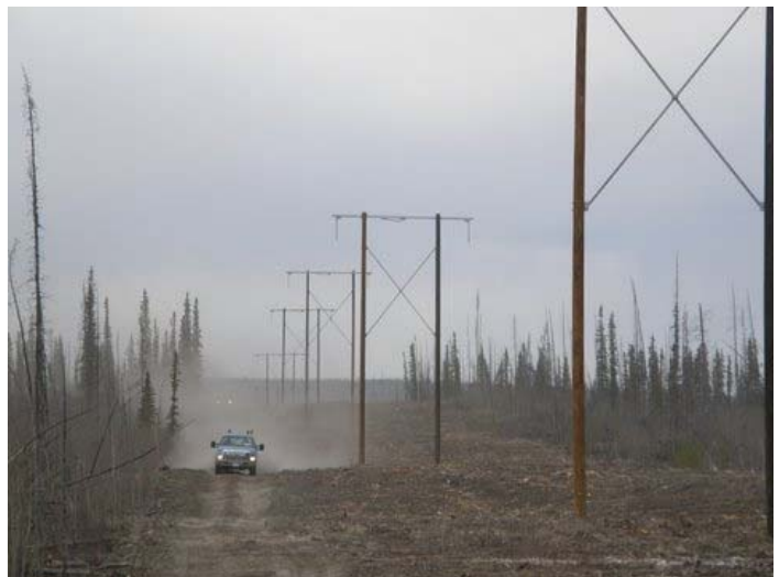
Pole structures on the Carmacks-Stewart line. Photo: Valard Construction
