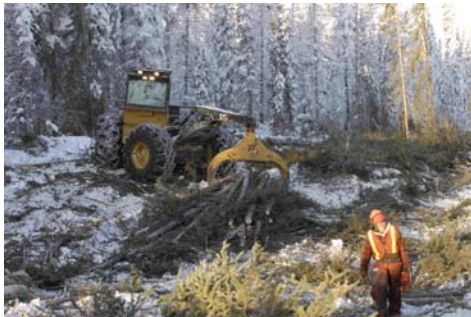
Clearing work on the Carmacks-Stewart line. Photo: Derek Crowe
