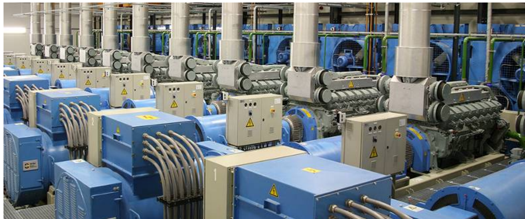
Figure 2. DRUPS Installation (Courtesy: Hitec Power Protection)
