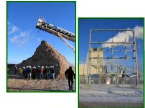
Dapp Power Plant Dapp, Alberta
