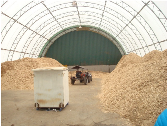
Figure C3: Fuel Storage Interior
