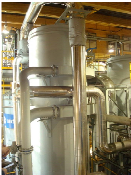
Figure N11: Thermal Oxidizer
