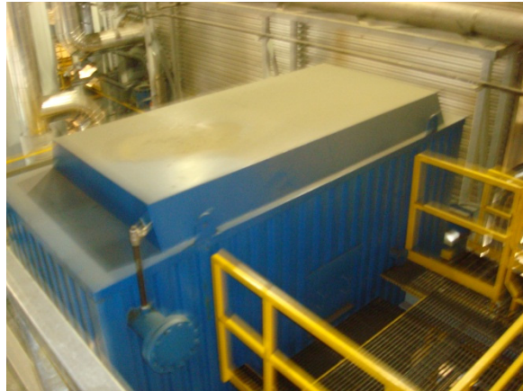
Figure N14: Electrostatic Precipitator
