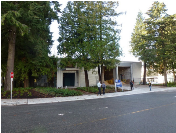
Figure N1: Building Exterior
